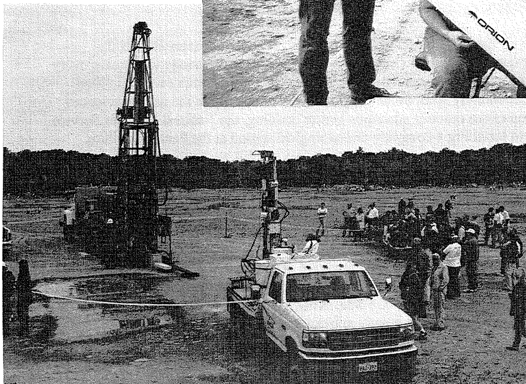
Figure 9. Maxim Technologies, Inc. demonstrating drilling & coring procedures on Earth Science Day. The drill rig is in the back- ground and a direct push rig in the fore- ground.
